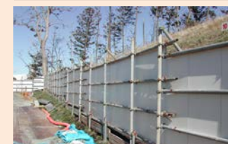
Temporary fence for
