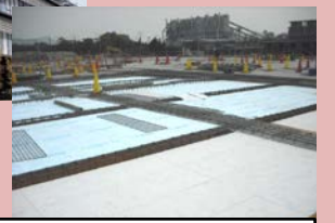
Concrete forms at construction site
