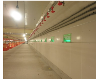
NF4 on ceiling, walls (chicken house)
