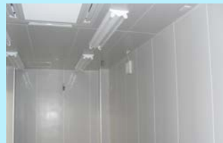
Interior wall of fish processing plant
