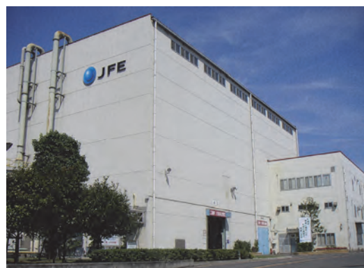
Fukuyama Division Fukuyama Recycling Plant
